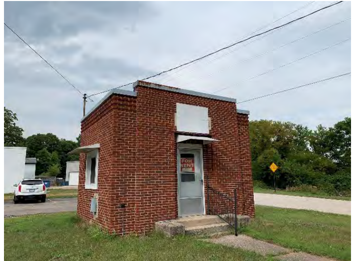
Potential Building for Tourism Reuse- Equipment Rental
